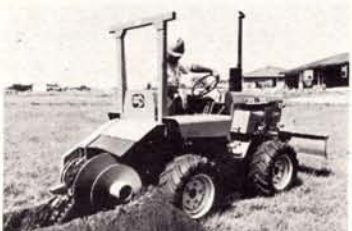
Single-auger digging assembly.
